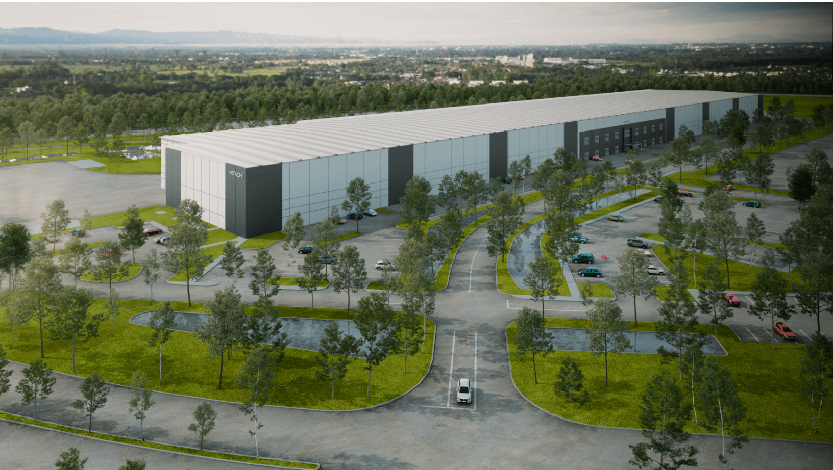
CGI of the Final Design for the New Maryland Factory
